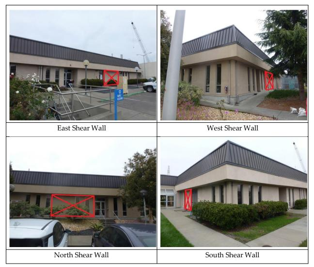
Figure 6: North Lab Addition – New Shear Wall Locations
