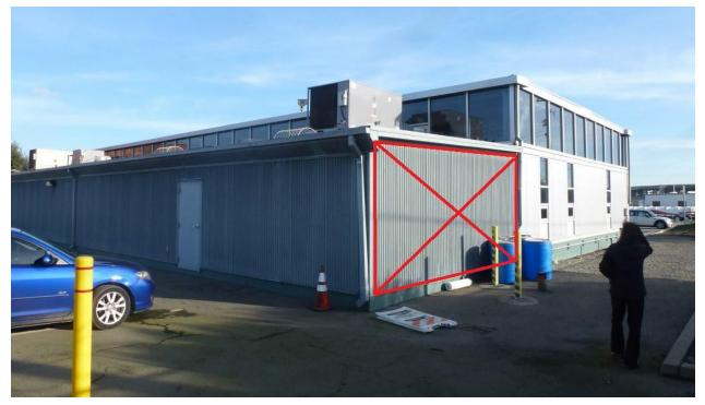
Figure 6: Field Services Building – Shear Wall at Line 1
