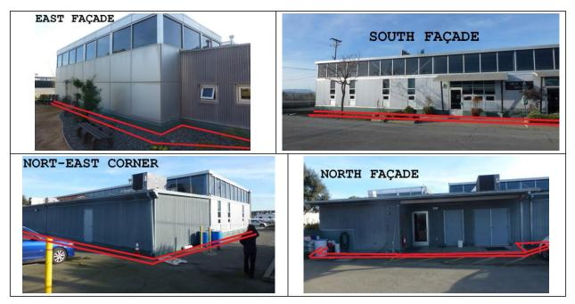
Figure 8: Field Services Building – Foundation Retrofit
