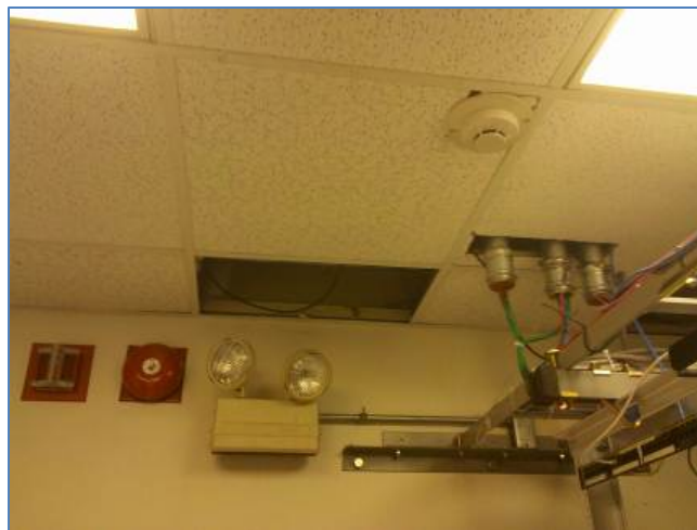
Figure 3. Detector and Notification Equipment
