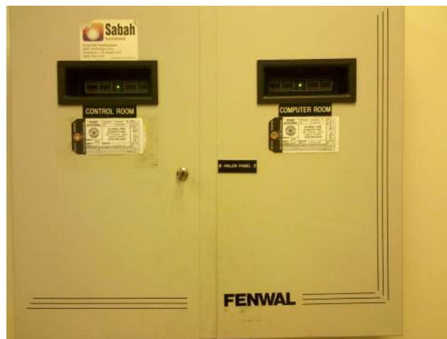
Figure 16. Fenwal Control Units for both Ops Control and Computer Rooms (located in Computer Room)
