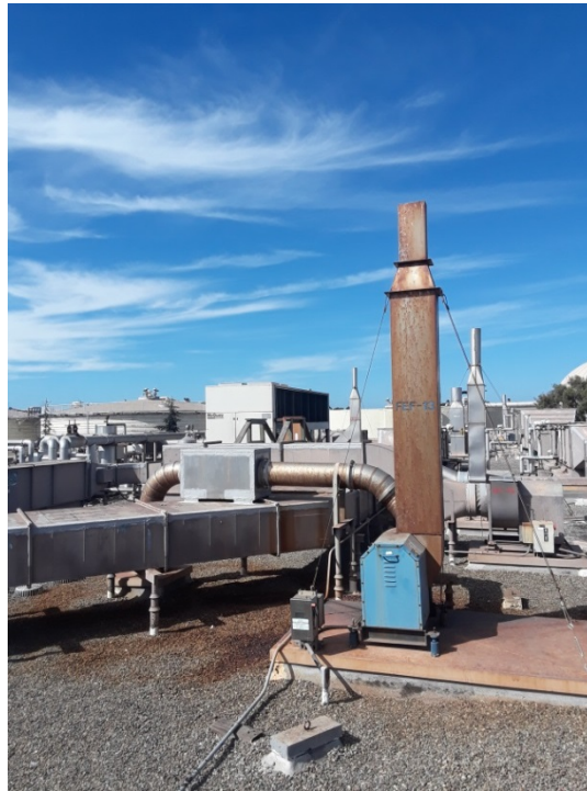
Figure 4: Corroded Fume Hood Exhaust Vents
