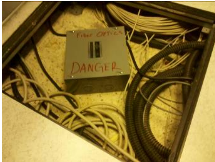
Figure 8. Sub-floor Debris and Cabling
