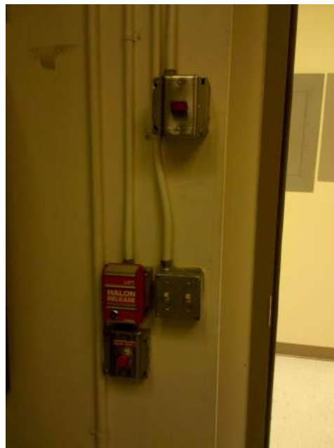
Figure 5. Halon Manual Release and Abort
