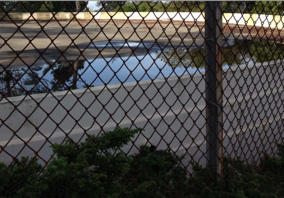
Ponding on Roof
