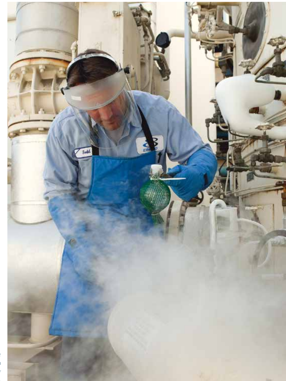
A wastewater plant operator collects a sample of liquid oxygen. EBMUD's pure oxygen production facility is used in the secondary treatment phase of wastewater treatment.
