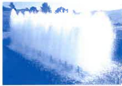
Aeration, shown at the Sobrante water treatment plant, consists of spraying water to allow it to release gases. This process improves the taste and odor of the water.
