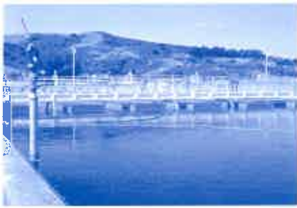
Sedimentation basins (the one shown is part of the San Pablo water treatment plant) allow heavy clumps of alum combined with dirt to settle to the bottom.
