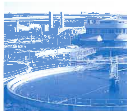
The center of operations of EBMUD's Wastewater Treatment plant is located in Oakland, at the foot of the Bay Bridge.
