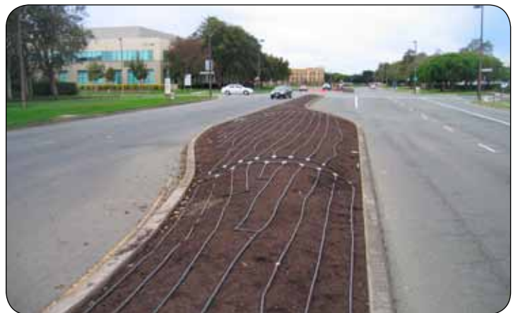
In-line drip irrigation was installed.
