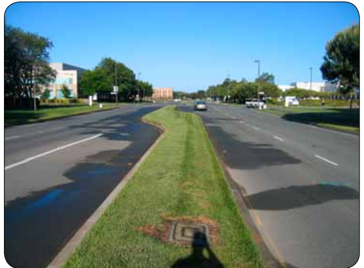
Before: Median with grass showing irrigation overspray.
