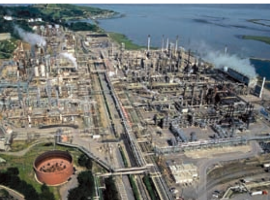
The Chevron Refinery in Richmond is EBMUD's largest user of potable and recycled water.
