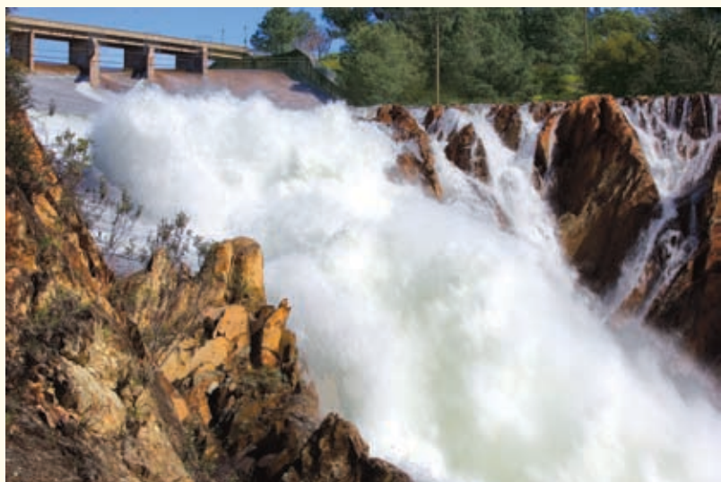
Pardee Reservoir spillway overflow from heavy 2006 rainfall and snowmelt.
