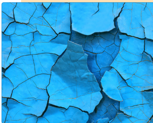
Lead was used in house paint until 1978, and the older the home, the more lead in the paint. (Source: Contra Costa Health Services)
