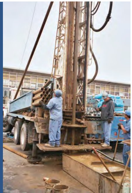
Drilling operation for nested monitoring well
