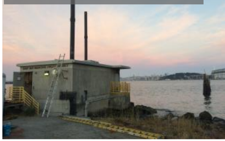
Outfall Transition Structure
