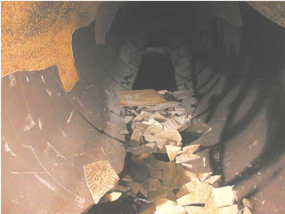
Delaminated lining accumulated on pipe invert
