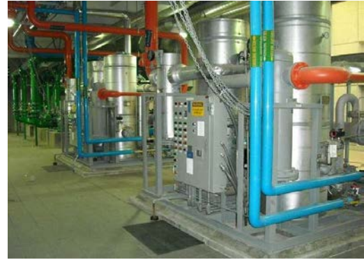
Water Treatment Plant Ozone System
