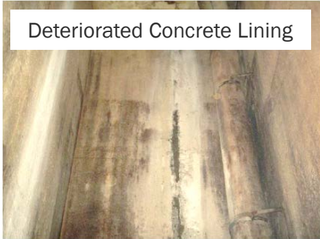
Concrete Support Corrosion
