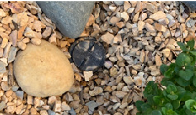
Sprinkler system capped
