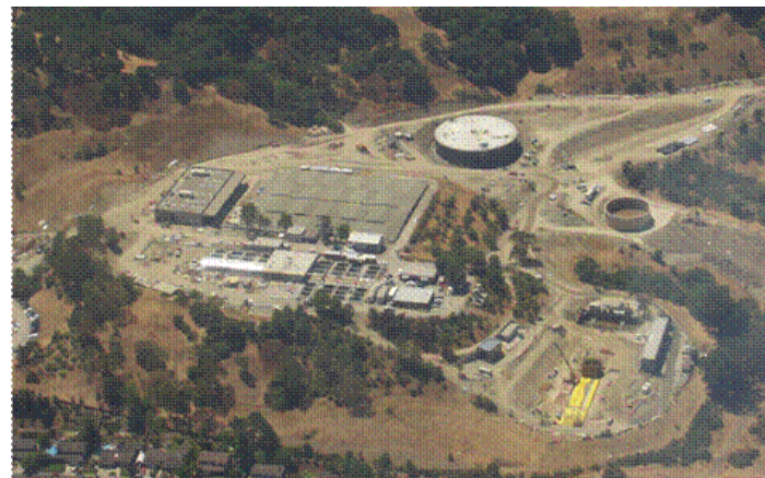
Walnut Creek Treatment Plant
