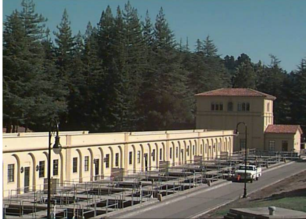
Orinda Treatment Plant
