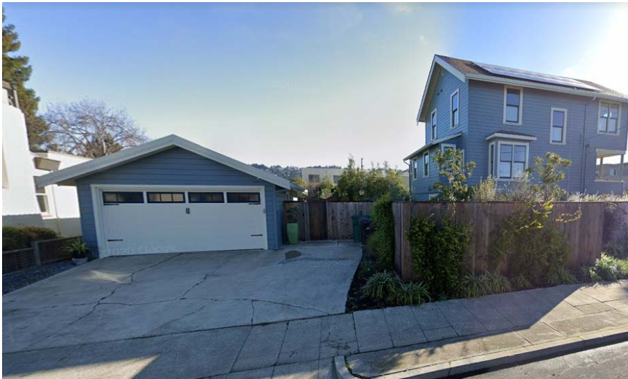
Before as garage
