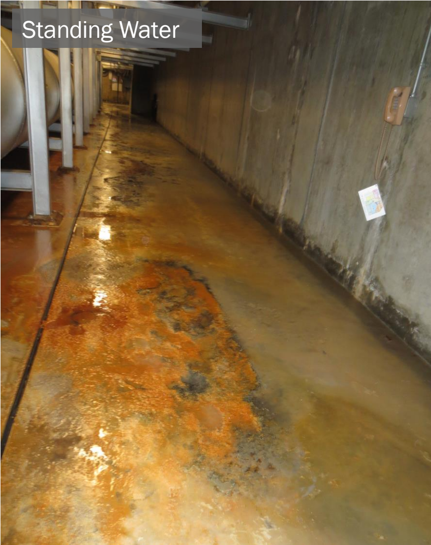
Leaking Penetrations
