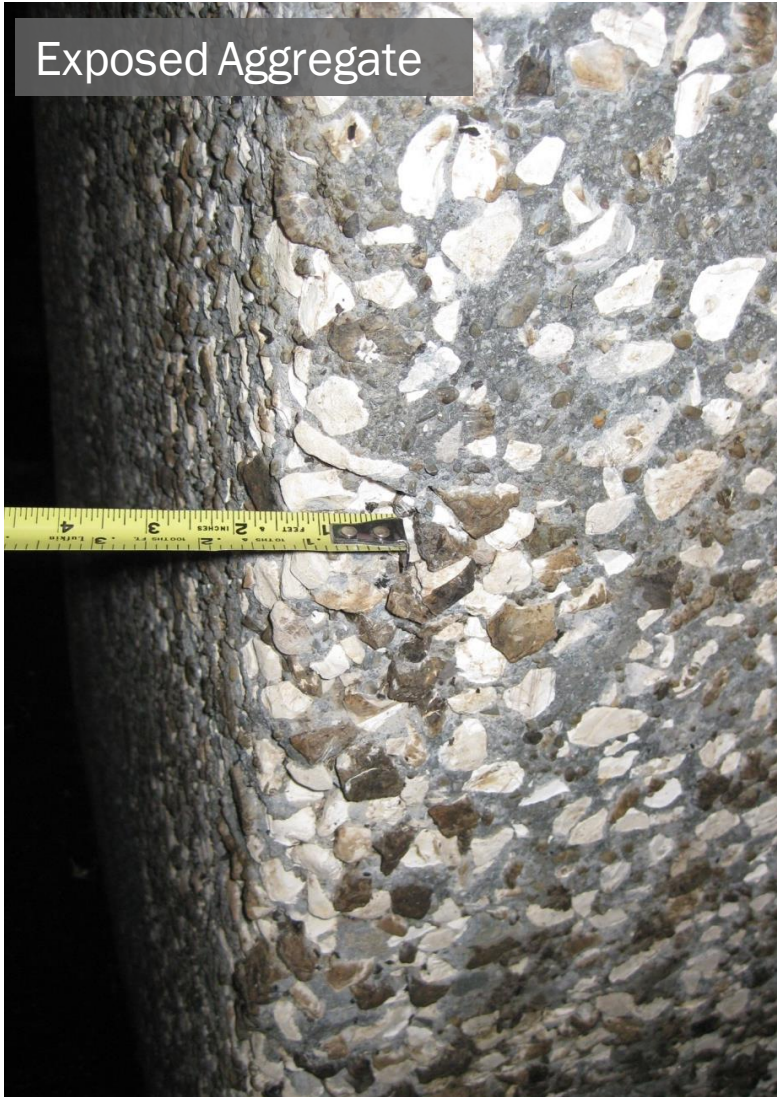
Exposed Aggregate & Patchwork
