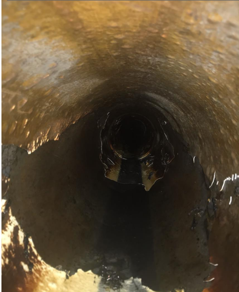
Deteriorated Lining Inside Pipe and Digester
