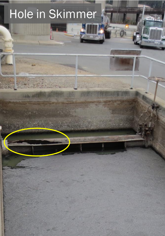
Corroded Metal
