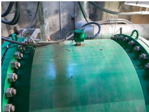
48" Effluent No. 1 Mag Meter
