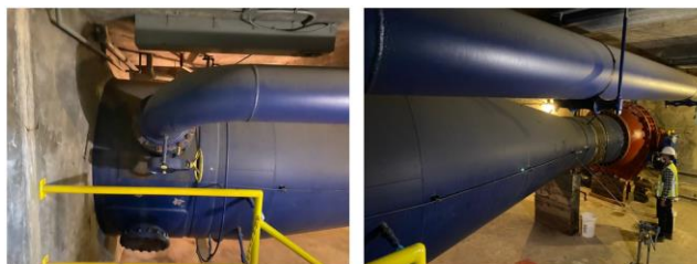
84" La Honda Venturi Meter located inside South end of Maloney Pumping Plant
