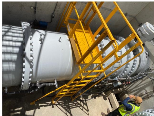
54" Effluent Pipeline Vault – Dall Flow Tube Meter Location
