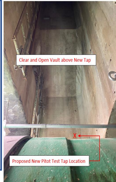
New Phase 1 Pitot Test Tap Location – 4' upstream of existing Mag Meter (proposed)
