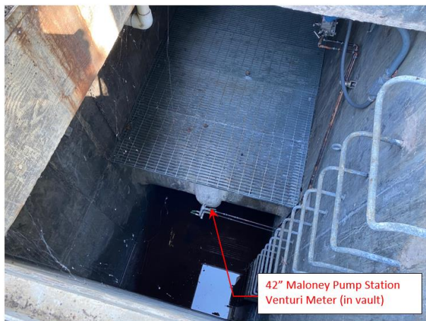
Maloney Pumping Plant Meter (located in vault just north of pumping plant building)
