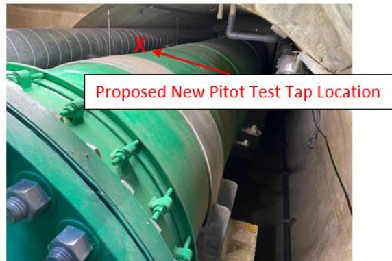
48" Effluent Pipeline upstream from Mag Meter
