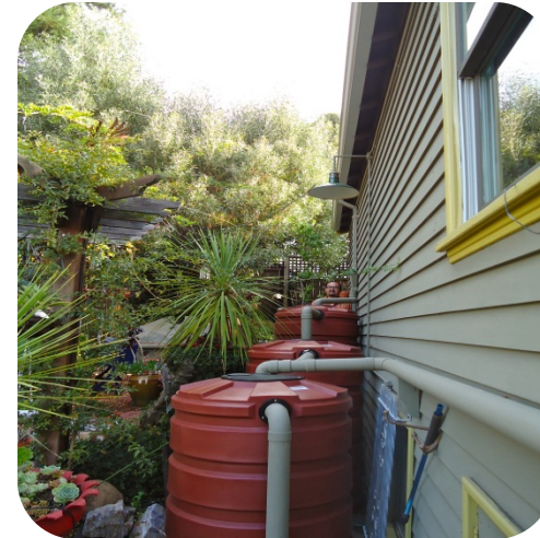
Daisy chained system of 205 gallon barrels Courtesy of The City of Oakland
