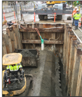
Pit #3: Preparing for removal of top of interceptor
