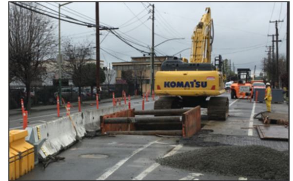
Pit #2: Installing shoring
