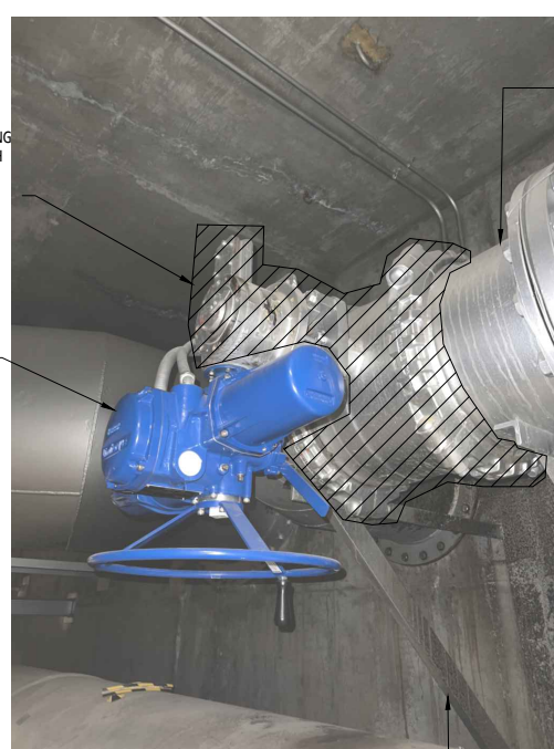
EXISTING 18" BFV W/ ELECTRIC OPERATOR FOR RAS TO REACTOR 5
