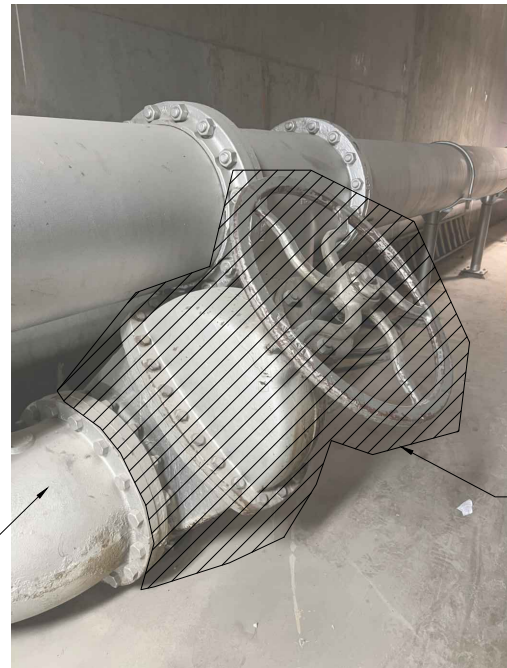
EXISTING 18" GATE VALVE W/ MANUAL OPERATOR FOR REACTOR 5 DRAIN
