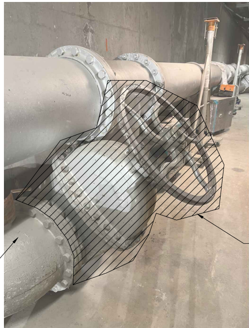
EXISTING 18" GATE VALVE W/ MANUAL OPERATOR FOR REACTOR 6 DRAIN
