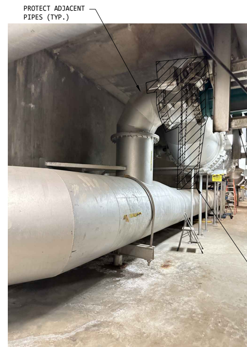
EXISTING 30" BFV W/ MANUAL OPERATOR CONNECTING RAS A & B
