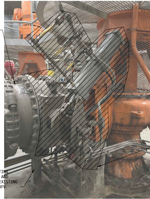
EXISTING 30" BFV W/ PNEUMATIC OPERATOR FOR RAS PUMP 3
