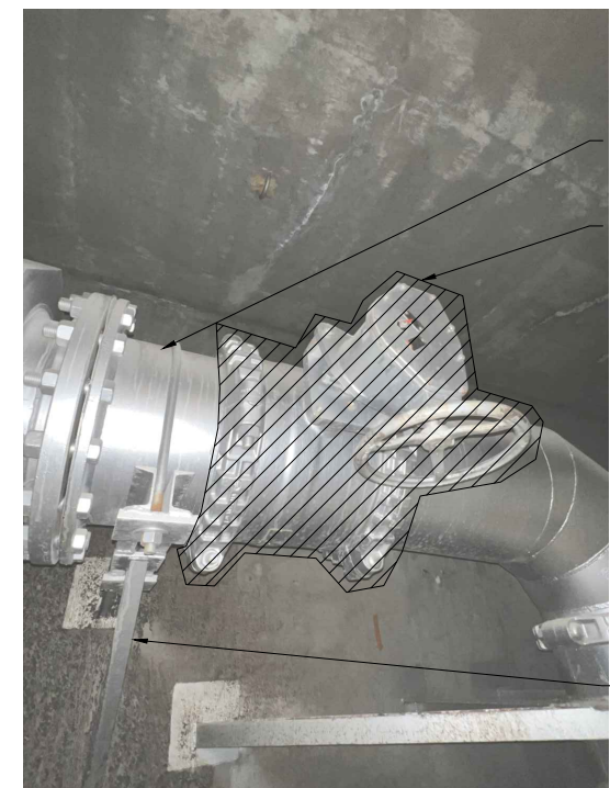
EXISTING 18" BFV W/ MANUAL OPERATOR FOR RAS TO REACTOR 5
