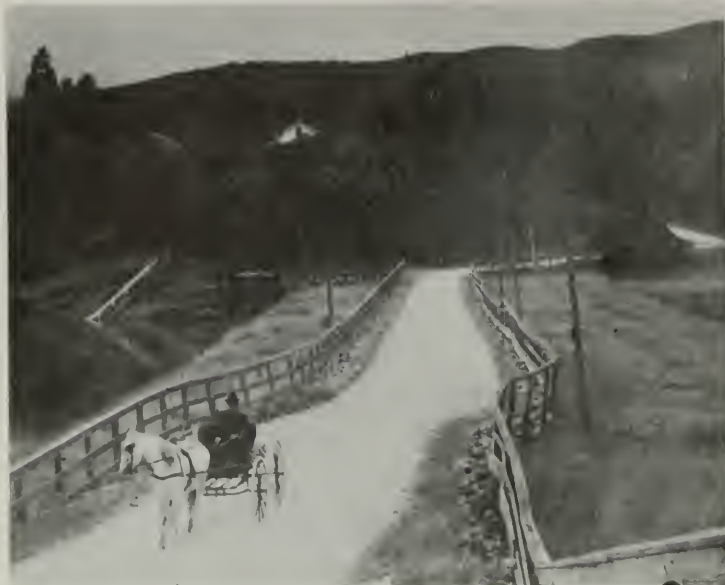
Photo 6. Causeway over Crystal Springs Reservoir offset during 1906 earthquake. Photograph courtesy of Bronner Library, Stanford University
