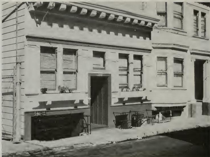
Photo 7. Building on Clara Street in San Francisco showing subsidence of filled ground over former swamp. Street and sidewalk have been raised to their original level by additional fill, and as a result the top of the garage door on left side of the house is only about 2 feet above the sidewalk.
