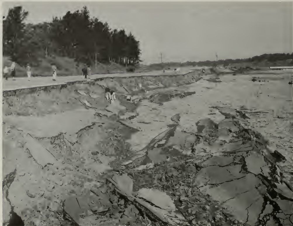
Photo 1. Earthquake damage to road on shore of Lake Merced, 1957. The landslides probably were caused by liquefaction during shaking of water-saturated sand.
