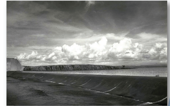
Camanche Spillway, February 1986 Peak Spill 1,630 cfs
