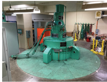
Current Condition (Unit No. 3)
