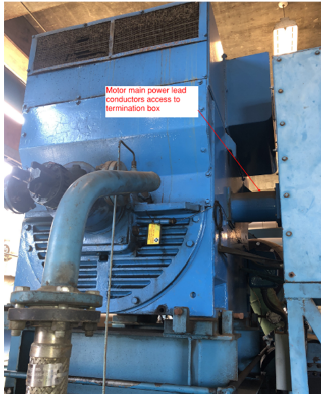
FIGURE 1 MAC 1-2 MOTOR POWER LEADS
