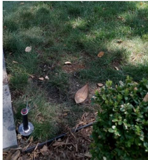
After- Irrigation zone watered with high-efficiency rotating nozzles.
