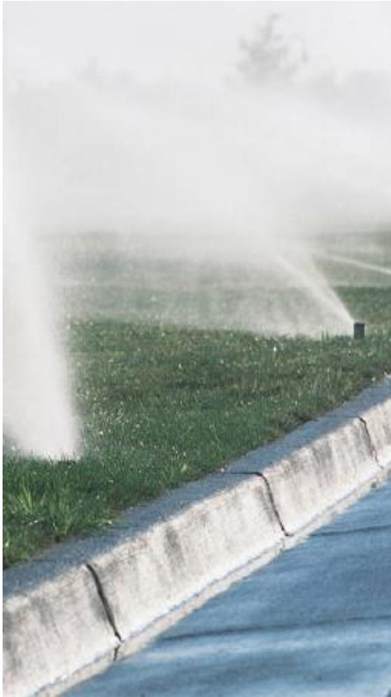
Before- Irrigation zone watered with inefficient fixed spray sprinklers that are causing misting, overspray and runoff.
