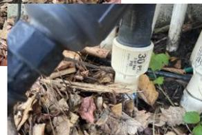
Drip pressure regulator and filter components
