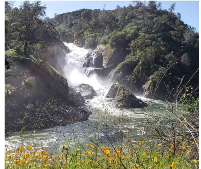
Downstream of Pardee Spillway
