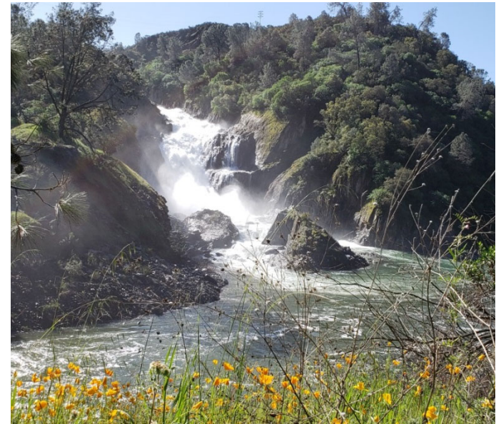
Downstream of Pardee Spillway
