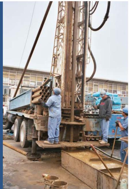
Drilling operation for nested monitoring well
