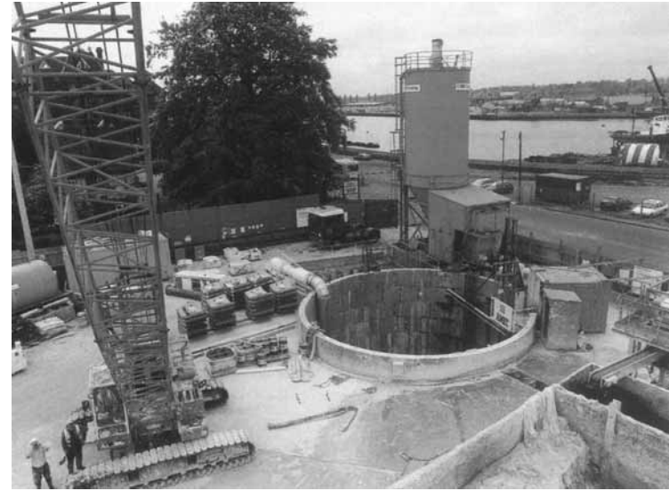
TYPICAL TUNNEL ENTRY SHAFT CONSTRUCTION SITE
