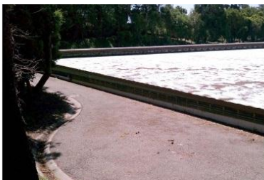
10 Maintenance access roadway
