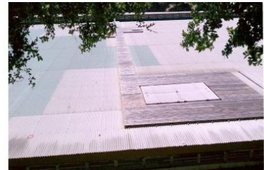
6 Roof view from homes to the north
