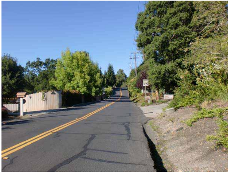
1. Looking northeast from Miner Road and Lombardy Lane intersection.
