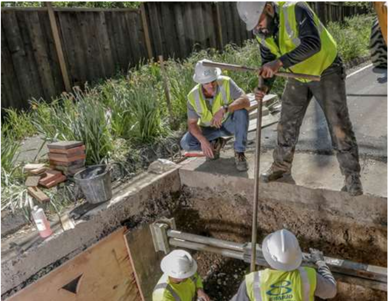
EBMUD work crew installing pipeline in the community.
