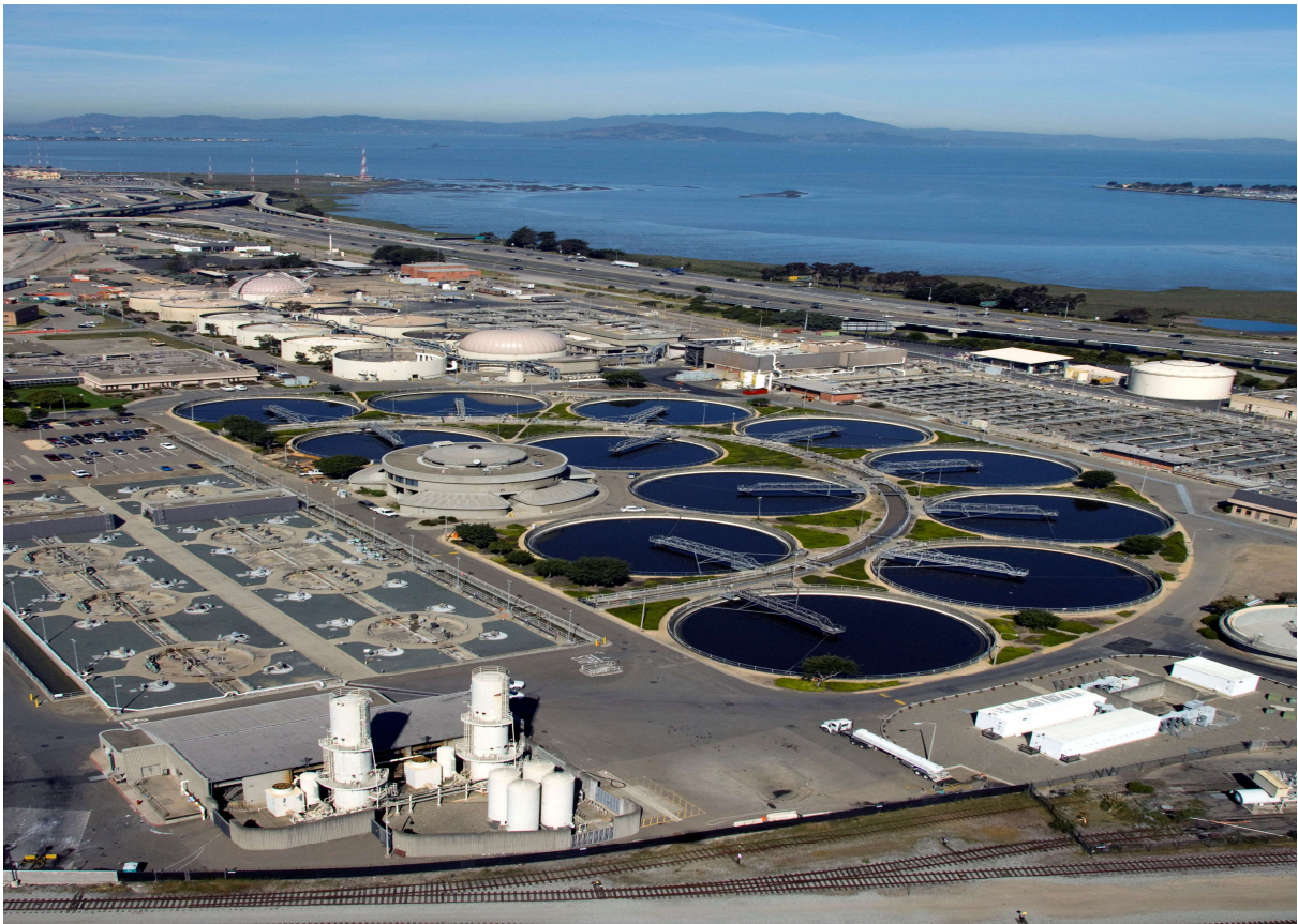
Main Wastewater Treatment Plant
