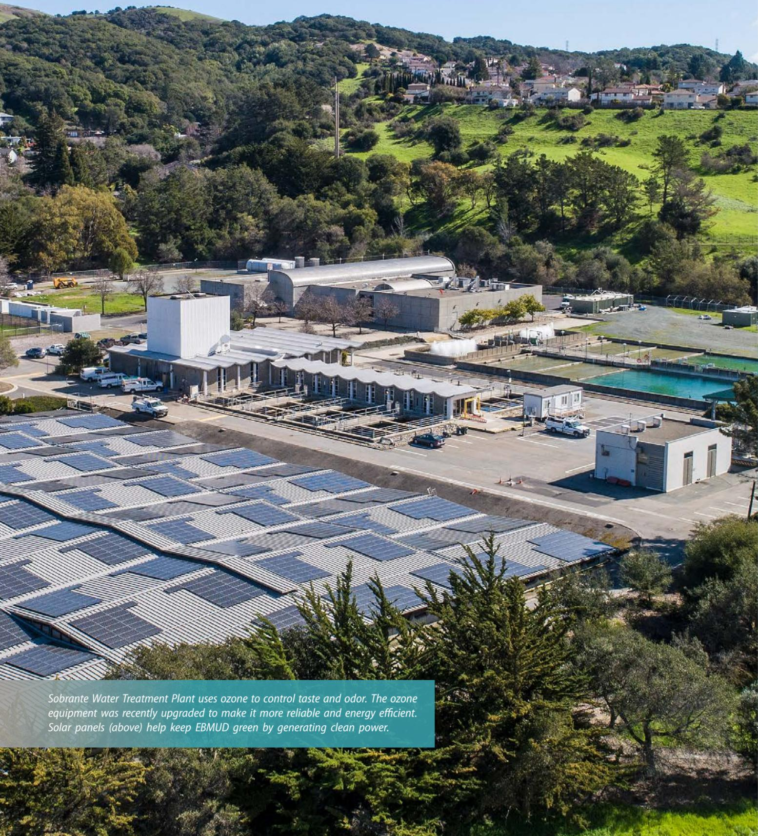
Sobrante Water Treatment Plant uses ozone to control taste and odor. The ozone equipment was recently upgraded to make it more reliable and energy efficient. Solar panels (above) help keep EBMUD green by generating clean power.
