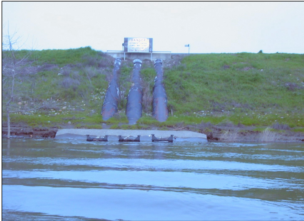
Photograph 1. Typical Riverbank Downstream of Proposed Structure
