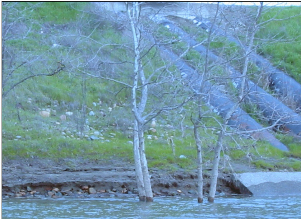
Photograph 2. Close up View of Outfall Structure Shown in Photograph 1.
