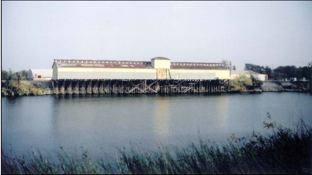
Photo 8. Looking across the Sacramento River at the riverside dock warehouse in the town of Hood. Note that this structure is relatively similar in architectural massing, proportion, and scale to the proposed intake facility. This structure is approximately 150 feet in length, 35 feet in width, and 30 feet in height.
