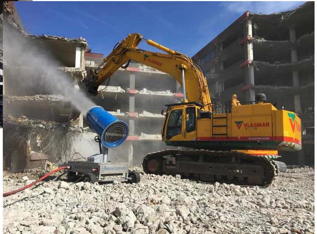
Machine wetting of demolition debris 24
