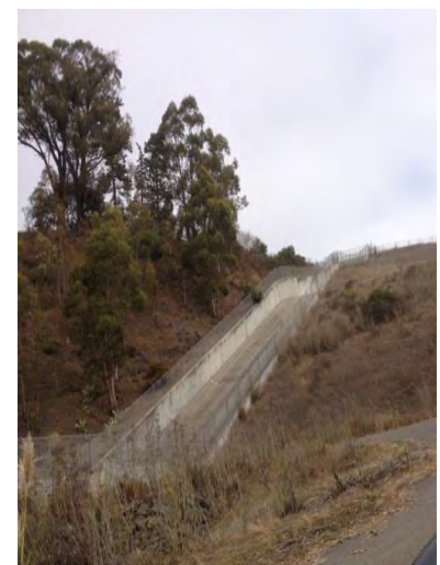
Photo 3.2-11: Chabot Dam Toe, looking east
