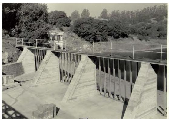
New concrete trashrack structure at Spillway No. 1, 1933 (Source: EBMUD)
