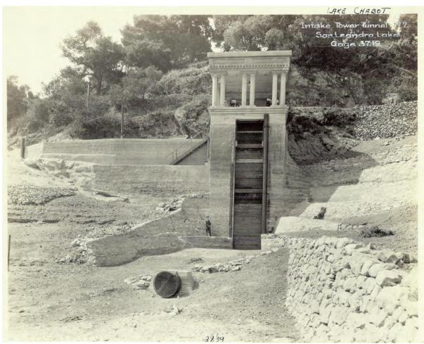
Tunnel No. 2 Intake Tower, circa 1924. (Note circular pipe inlet at lower center and rubblerock wall at upper right.) (*Source: EBMUD*)
