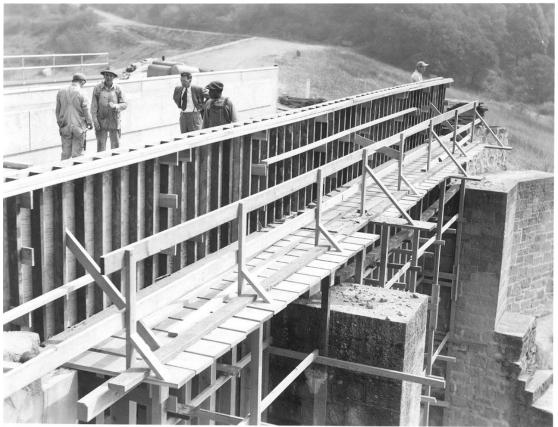
Construction of New Pedestrian Bridge over original masonry weir at Spillway No. 1, 1933 (Source: EBMUD)
