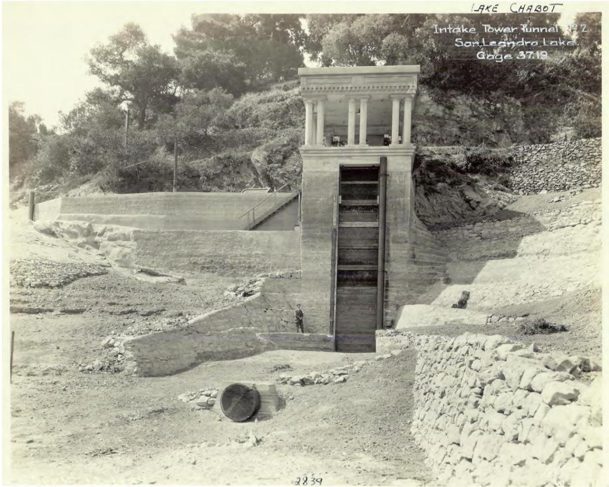
Tunnel No. 2 Intake Tower, circa 1924. (Note circular pipe inlet at lower center and rubble-rock wall at upper right.)
