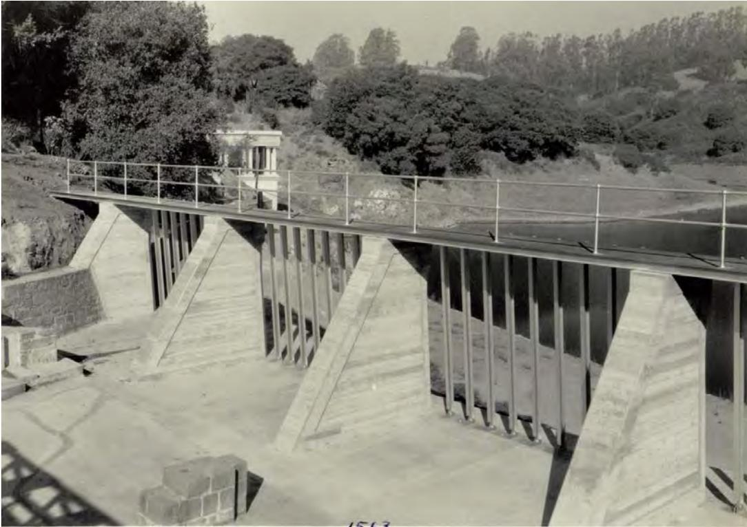
New concrete trashrack structure at Spillway No. 1, 1933
