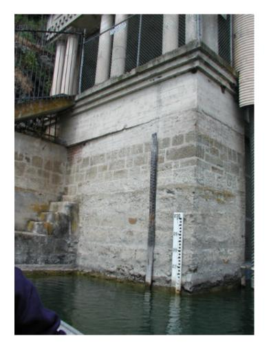
SOUTH FACE CONCRETE FLOOR AND PERIMETER OVER BRICK OVER DRESSED STONE OVER STONE
