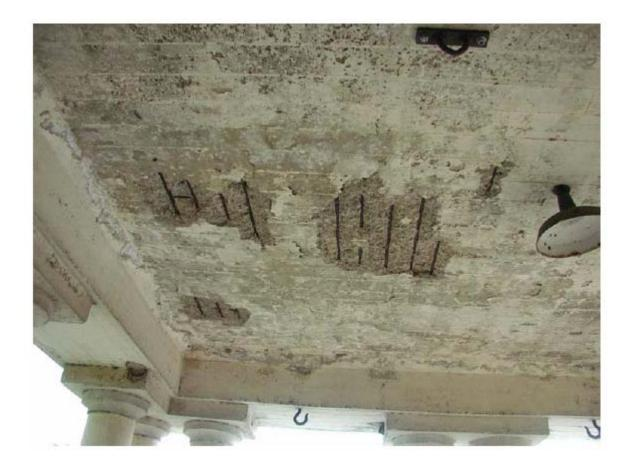
**Concrete Spalling at Pavilion Roof**
