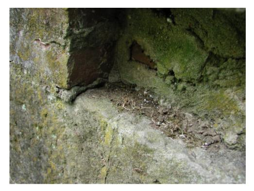
COLLAR JOINT AT REMOVED BRICK
