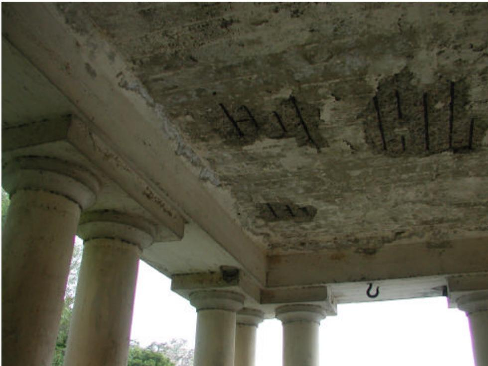
SPALLING AND RUSTING AT ROOF
