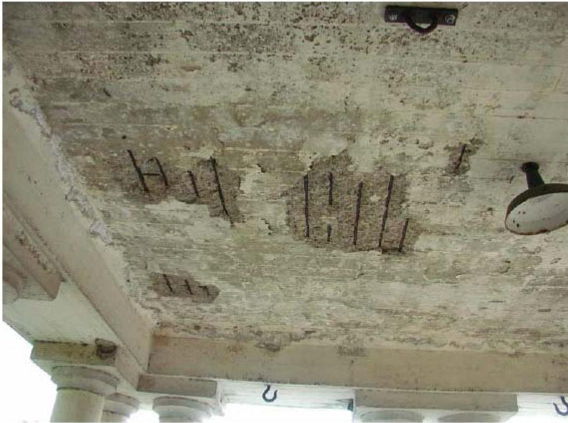
**Concrete Spalling at Pavilion Roof**
