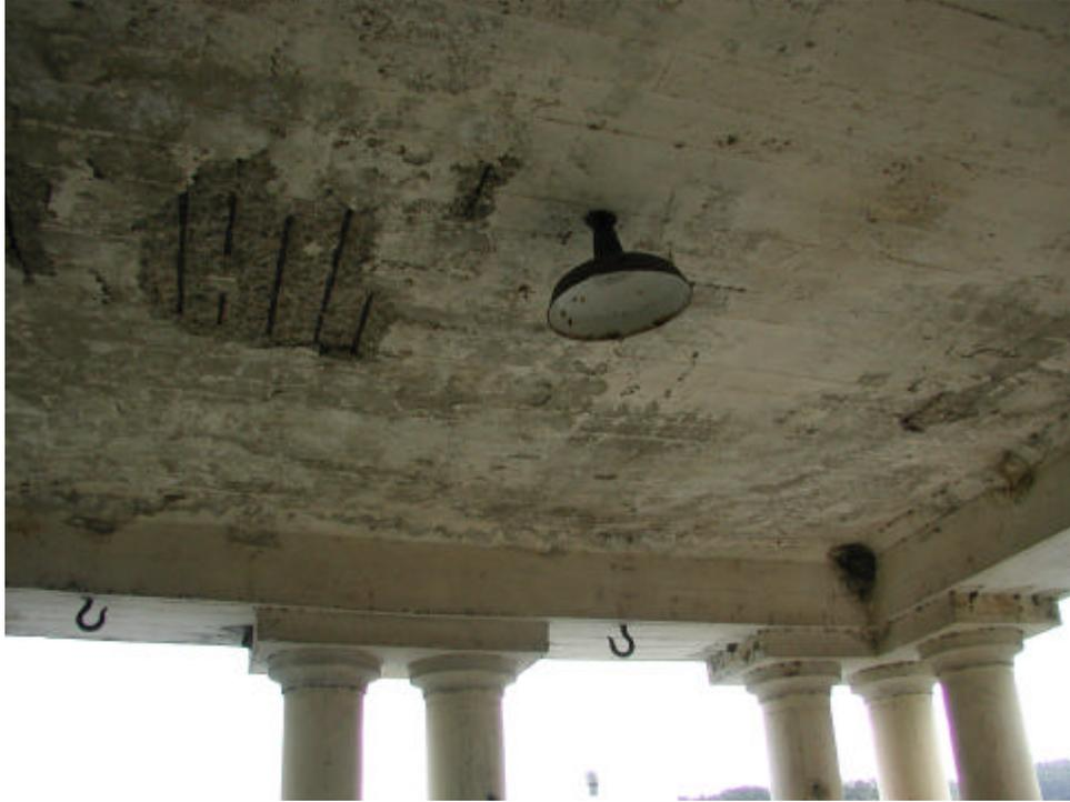
SPALLING AND RUSTING AT ROOF
