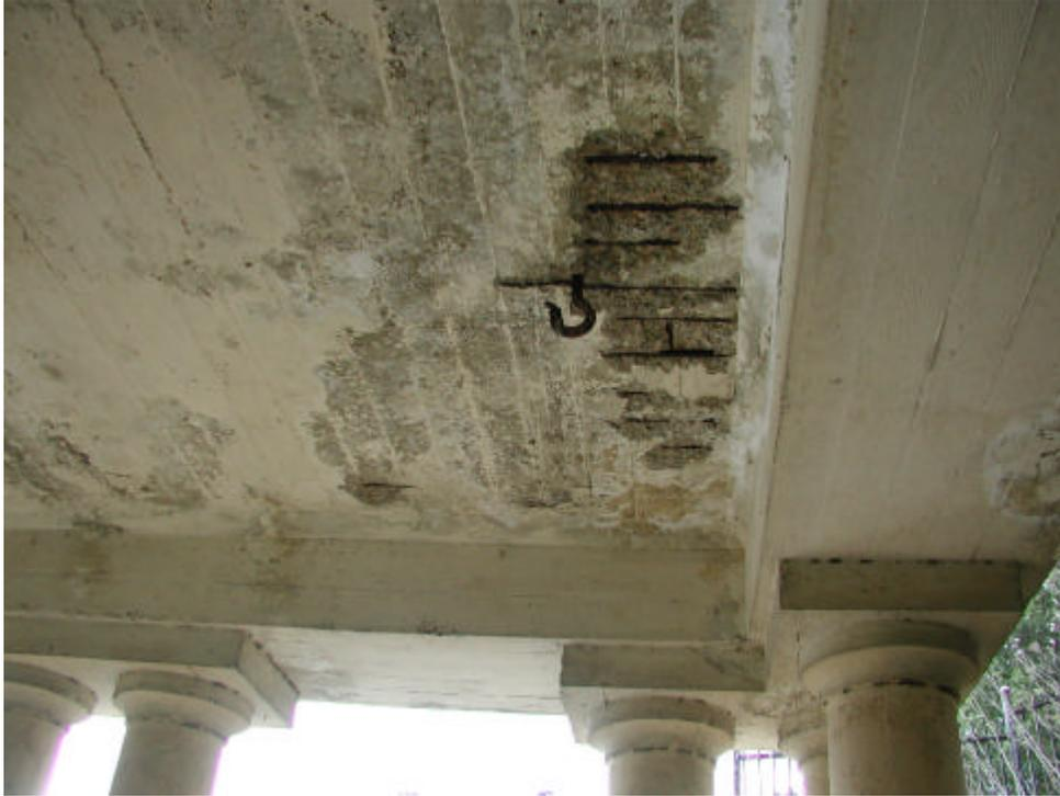
SPALLING AND RUSTING AT ROOF
