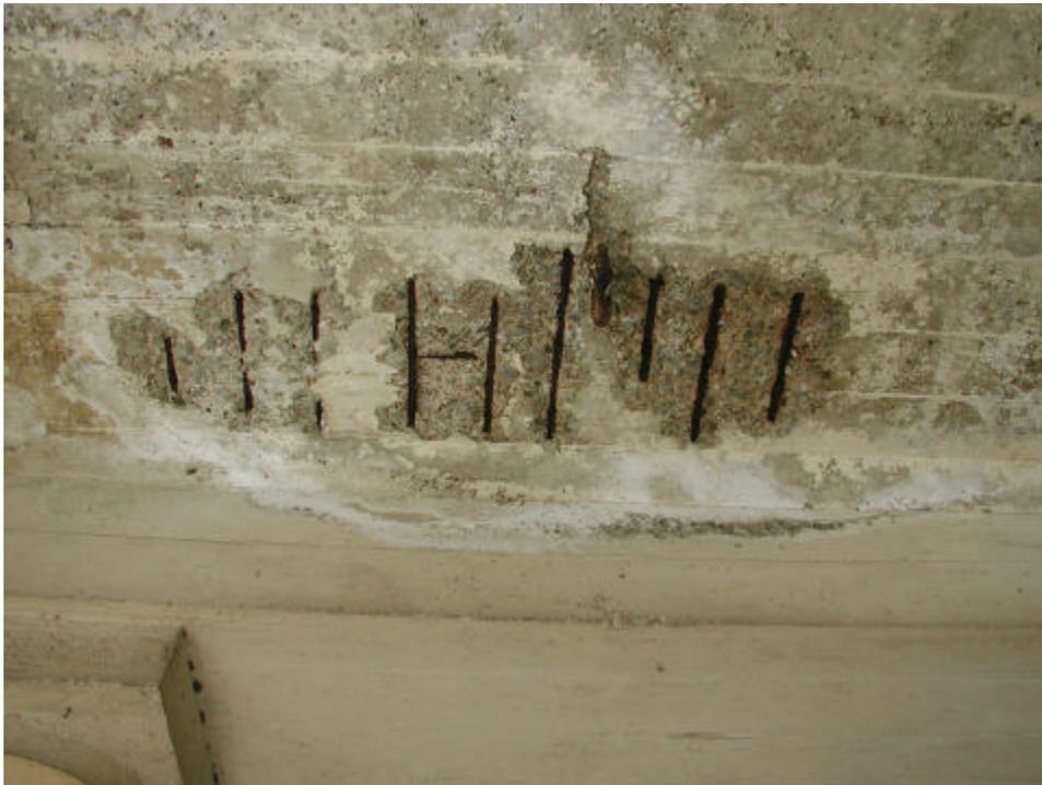
SPALLING AND RUSTING AT ROOF
