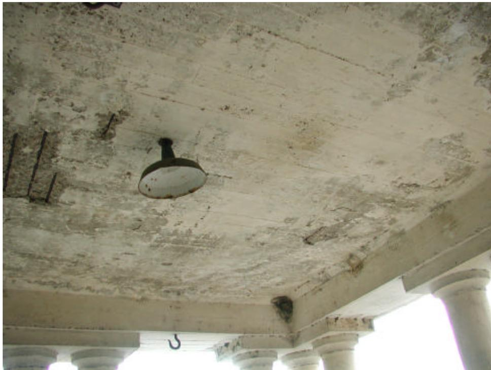
SPALLING AND RUSTING AT ROOF
