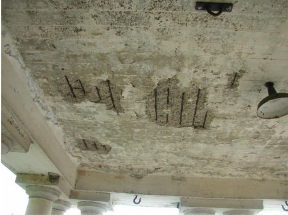
SPALLING AND RUSTING AT ROOF
