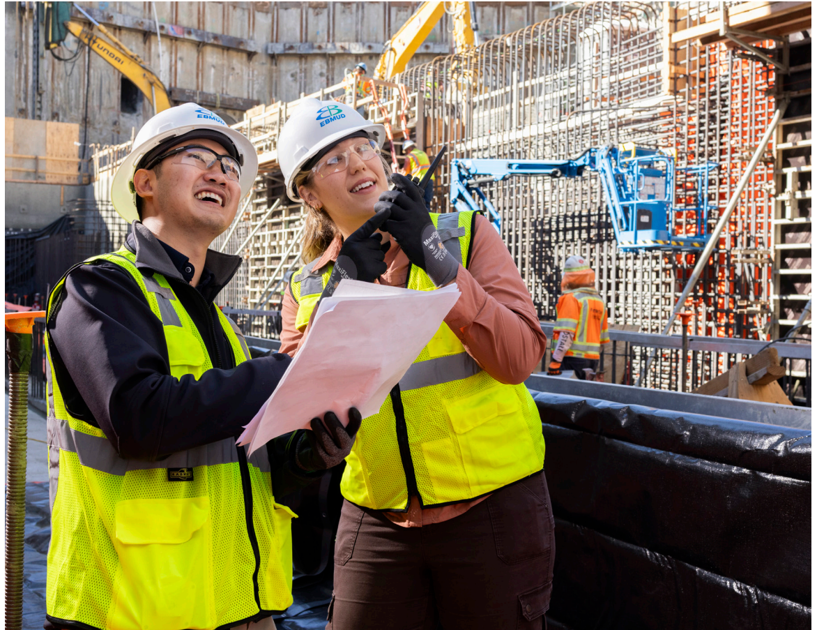
Above EBMUD project engineers review plans during construction.
