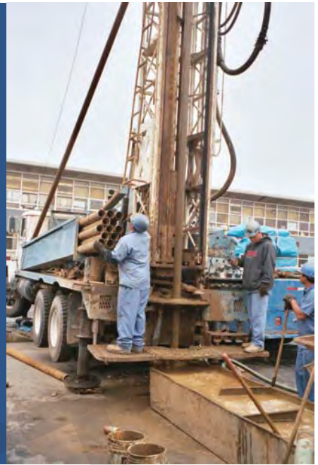
Drilling operation for nested monitoring well
