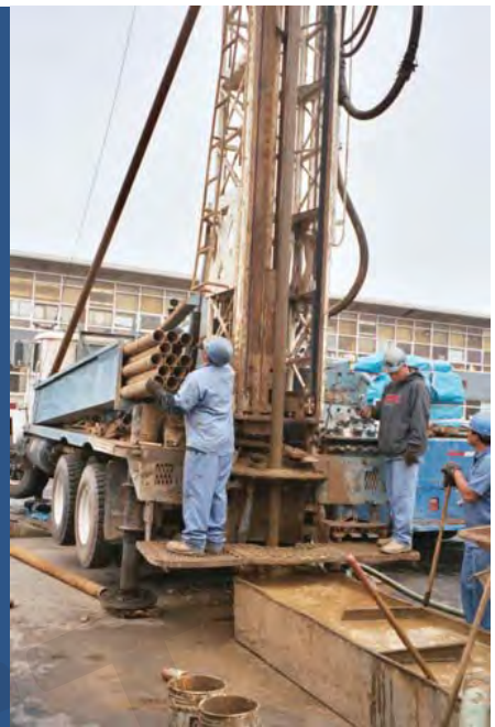
Drilling operation for nested monitoring well
