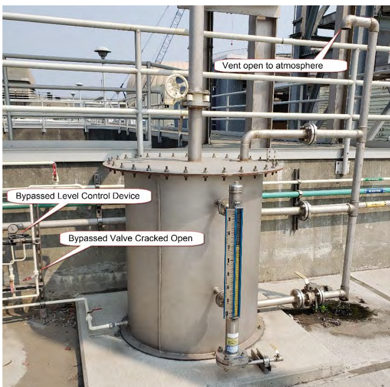
Figure 38 - Condensate Drip Trap Observations
