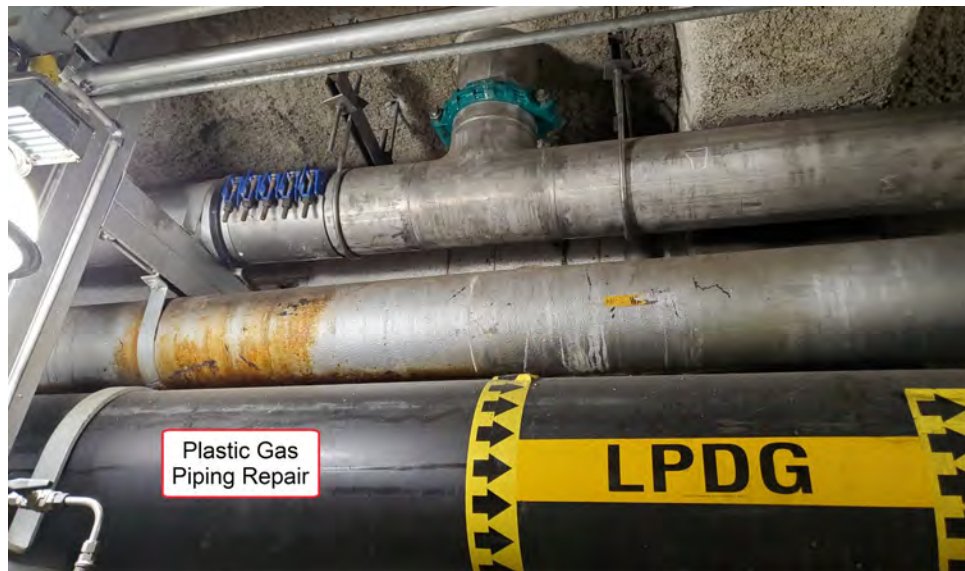
Figure 1: LPDG Gas Piping
