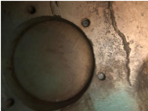
Left bank (exhaust side) flywheel side core plug viewed from bottom of bedplate through access holes, no signs of oil leak.
