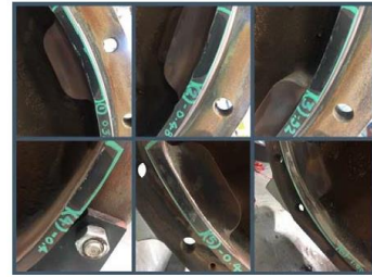
Fig. 4: Worn out hood clamping area.
