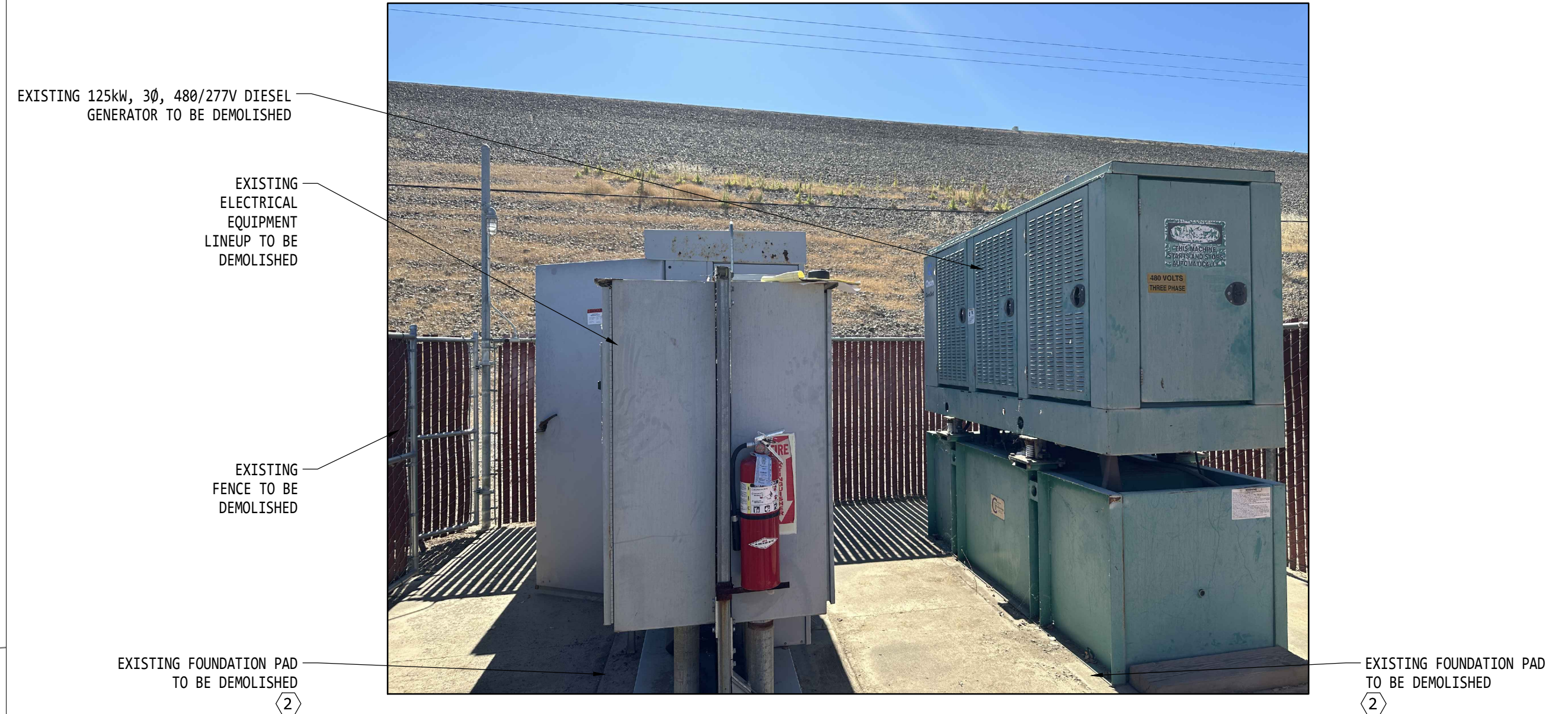
EXISTING SWITCHBOARD & GENERATOR NOT TO SCALE
