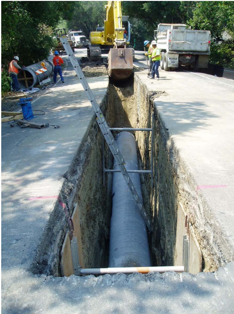
Installing Pipe in Roadway
