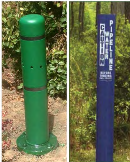
Figure 2-4: Air Valve Vent and Marker Post
