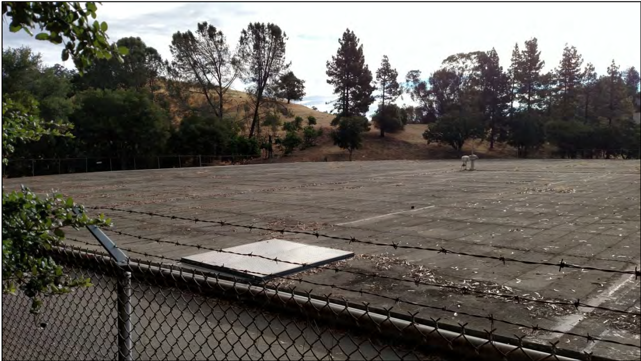
Photo 7: View NE, looking over the reservoir roof.
