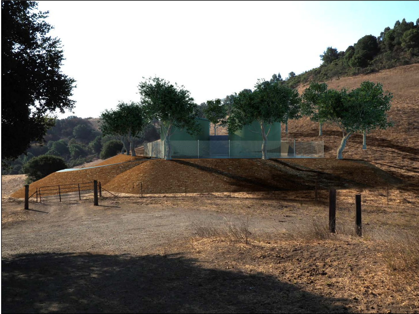
Figure 3.5b Simulated view from horse corral. This photo simulation of the new Dos Osos Reservoirs site shows the new dual reservoirs, retaining wall, security fencing, constructed earthen berms, and planted trees. The viewpoint is from a horse corral approximately 150 feet away from the site.
