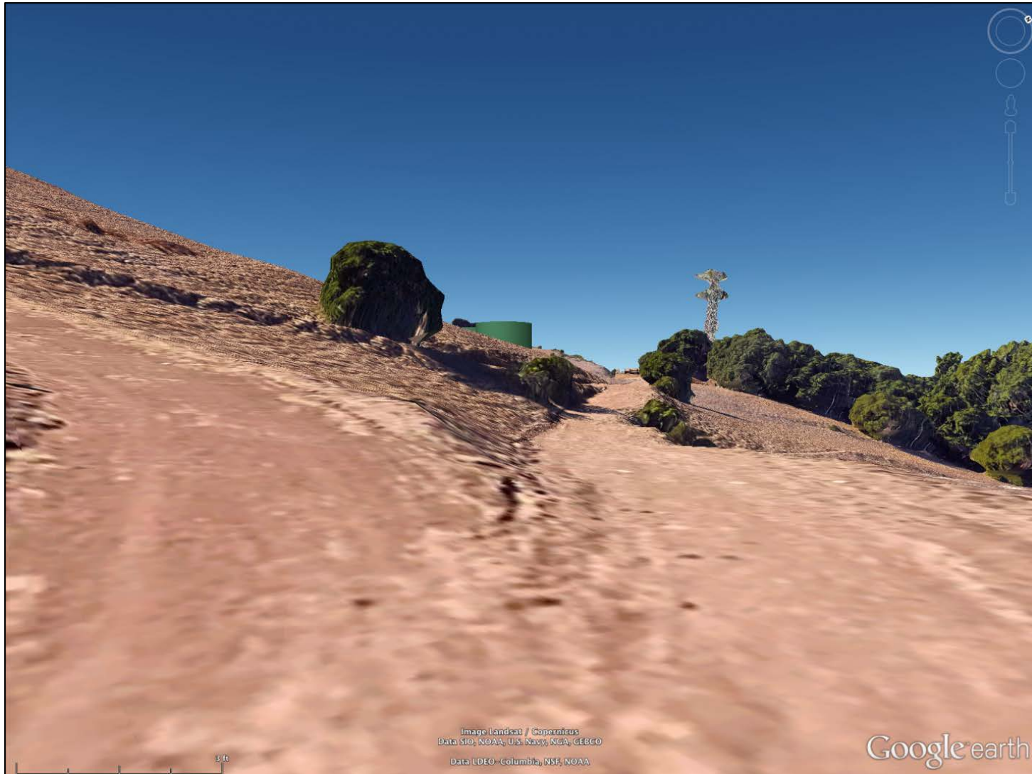
Figure 3.3 Simulated view from De La Veaga Trail. This visual simulation shows the view of the new Dos Osos Reservoirs from the closest point of the De La Veaga Trail, approximately 500 feet away from the reservoirs. The public trail continues to the left; the private fire access road is on the right.
